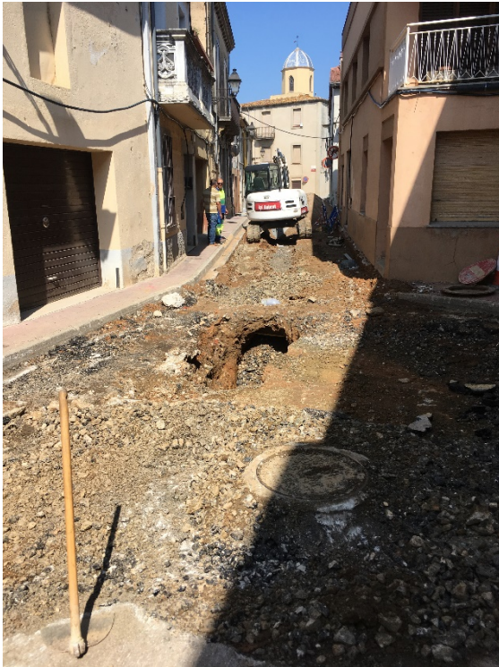
Enderroc total tram c. Girona- c. Roscada c. Roscada
